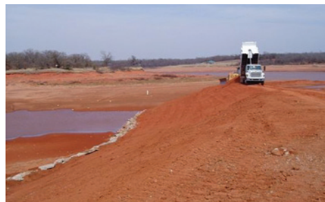
A new breakwater is under construction at Draper Lake.
